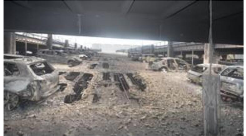
Figure 1. Reinforcement exposed by explosive spalling (left) and the fire-damaged concrete floor of the Liverpool Echo Arena parking garage (31.12.2017) (right)
